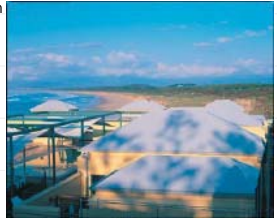
Steel roofing is now almost 100% Zincalume (zinc-aluminium alloy) coated, and combined with a proprietary paint coating for added appearance and durability. The zinc-aluminium alloy has excellent corrosion resistance for this application.
