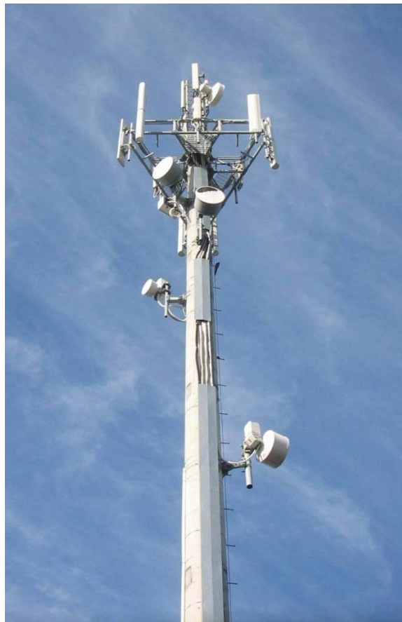
Fig. 1: Typical communication tower with antennas and headframe
