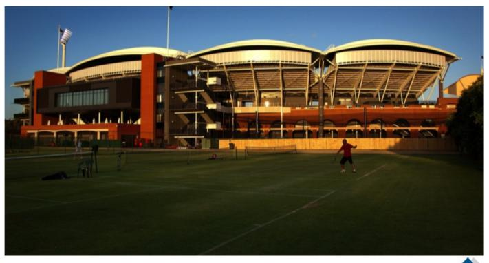
A critical component of improving patron amenity was improving the roof coverage from rain and for shading patrons from the sun. Coupled with this was an essential requirement for unobstructed views, necessitating a cantilevered steel roof solution. Aurecon undertook a multitude of design options to achieve these objectives.
