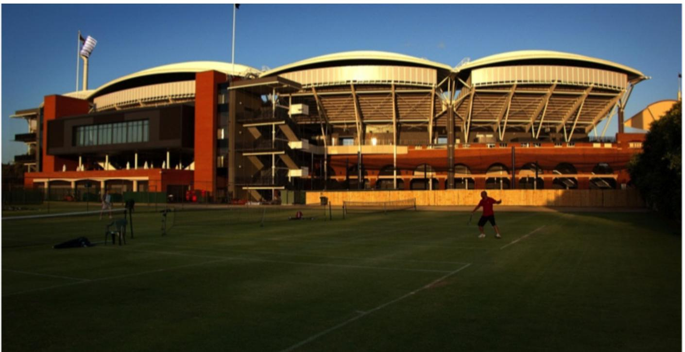
A critical component of improving patron amenity was improving the roof coverage from rain and for shading patrons from the sun. Coupled with this was an essential requirement for unobstructed views, necessitating a cantilevered steel roof solution. Aurecon undertook a multitude of design options to achieve these objectives.
