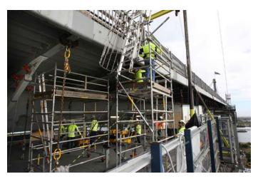
phistication with the design detailing. It was a requirement of the design that the detailing of fabricated elements were small and light enough that they could be lifted into the bridge through the manholes and transported along the inside of the bridge by hand.
