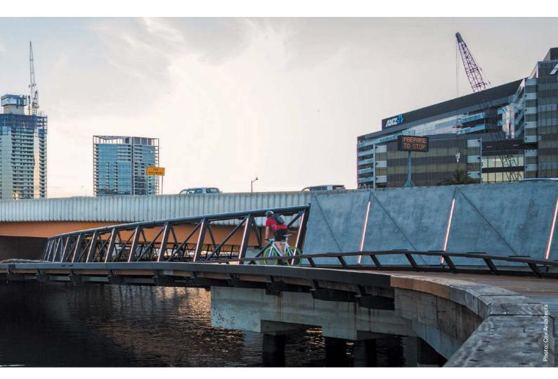
He said the structure is designed to be submerged during major flood events and to withstand log impact from debris floating down the river. The steelwork is coated with a high performance paint system.
