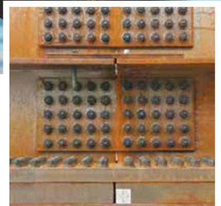
By facilitating steel-intensive bridgework, weathering steels open up a raft of structural benefits, including the base material's innate qualities, such as high strength-to-weight ratio, lower and variable structural depths, longer spans, splice connections for continuous spans, less demand on substructure design, rapid construction, fabrication off-site in controlled, automated workshops, and all steelwork being visible for inspection in the finished structure.
