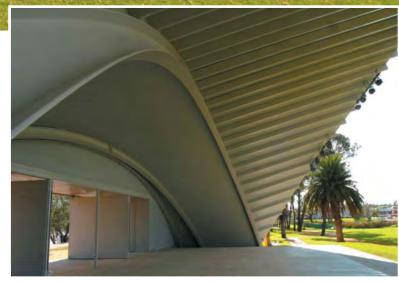
throughout from steel portal frame to cladding and an innovative steel fibre reinforced concrete slab. Sway portal frames were used at 21-metre centres with rafters spaced 10.5 metres apart. Exacta® purlins span the bays reducing conventional purlin weight over the entire warehouse area. Externally, COLORBOND® blades situated next to the office windows form a decorative façade and provide shading. Practical completion was achieved two weeks ahead of schedule.
