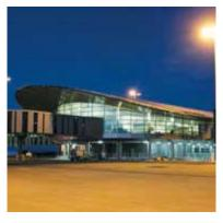
forms which were well considered to seamlessly integrate to the existing airport envelope. Using steel as the structural element enabled much of the work to be carried out away from the busy site. The judges considered the fit-for-purpose expansion to be an impressive feat of architecture and engineering and a tremendous asset to Perth Airport.
