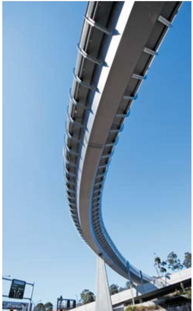
The Aurecon-engineered and steel-intensive Falcon Street Pedestrian and Cyclist Bridge that crosses 19 lanes of traffic with one span in Sydney
