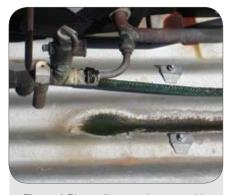
Figure 1 Bi-metallic corrosion caused by "copper-rich" water run-off
