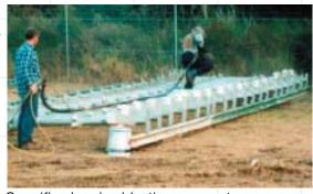
Specific abrasive blasting parameters are required when preparing galvanized surfaces for painting. The same techniques used for
