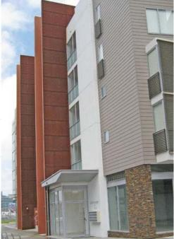
These architectural elements on a harbour-side building in Newcastle, NSW are fabricated from uncoated weathering steel.
