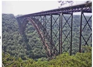
While not widely used in Australia, weathering steel has been used extensively in structural applications in the USA, with several thousand tonnes used on the New River Gorge Bridge in west Virginia.
