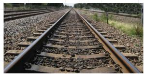
There are many instances where steel is used without a protective coating. Rail lines are a good example and have excellent durability in most Australian environments.
