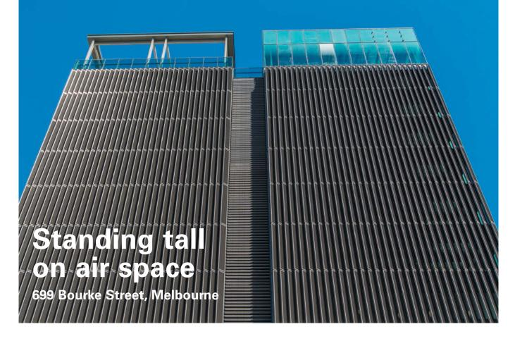
A lightweight steel frame has been adopted to seamlessly construct an office tower high above one of Australia's busiest railway hubs on a 24-metre high deck.
