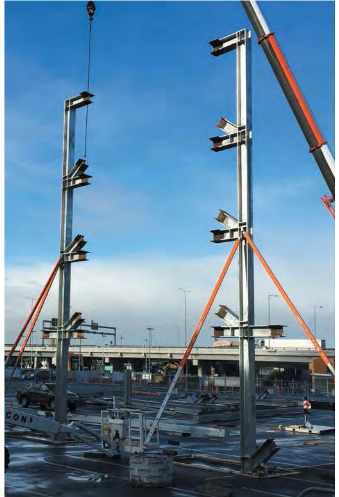
Starting up with the 13-metre high columns.
