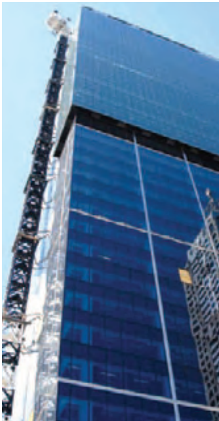
Extended glazing from floor to the underside of the slab above maximises the views and natural light penetration.
