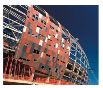
This design allowed the structural steel sub contractor to optimise the specially developed details which facilitated the transportation and lifting of the heavy steel elements. Bolted and hinged joints were designed to adjust the structure with jacks during erection ensuring a speedy and fluent sequence.
