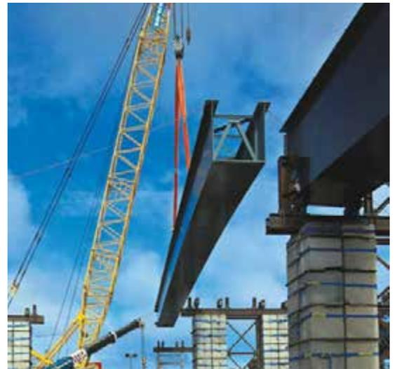
“Moving the finished girders around our site has been made possible and efficient through the adaptation of some steerable ‘jinker’ trailers we bought, hydraulic lifters installed under the deck as well as steering both ends and slew rings to enable turning under the girder.
