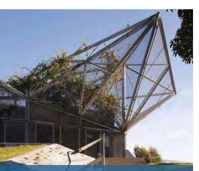
"He said that its landscaped roof garden is veiled by a steel canopy structure designed to support a variety of native climbing and fruiting plants as an interlocking, but self-supported element allowing for the future demounting and relocation of the structure."
