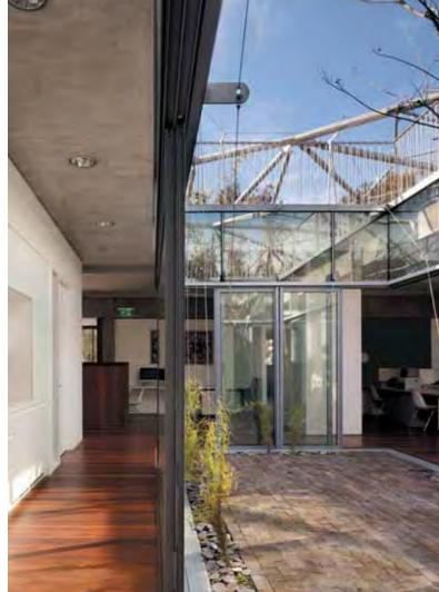
"The 'space frame' shape supplied by the architects meant that we had significant challenges in developing the mitre joints which were complex," he said. "And the fact that the frame was tubular added another degree of difficulty."
