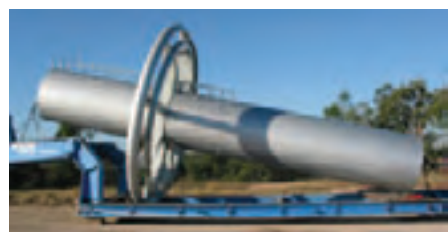
Individual mast units were prefixed off site before erection and installation.
