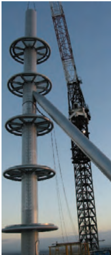
Nine units were installed to a series of meticulously planned lifts using the builder's tower crane.
