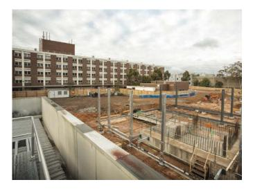
"Essentially it was a straight material substitution between concrete and steel. Obviously the structural detailing was different, but the basic form of the building was maintained and functionality and architecture was not compromised in any way."
