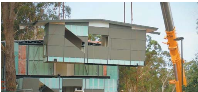
Modular accommodation unit being craned into place on CSU Student Accommodation, a project recently entered into the 2018 Australian Steel Institute's NSW and ACT Steel Excellence Awards. Photo: Intelligent Building Systems.
