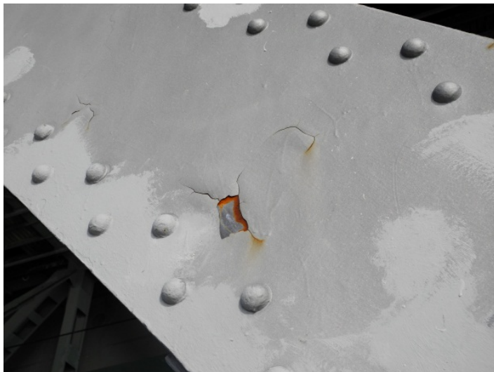
Figure 5.4: Example of damaged coatings – Auckland Harbour Bridge
