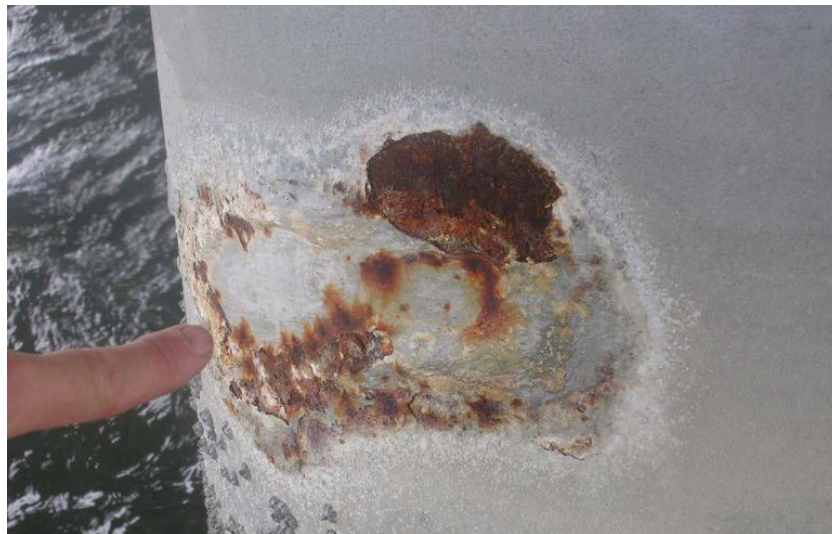
Figure 5.2: Failure of epoxy repair on TZA on Ahuriri Bypass bridge piling
