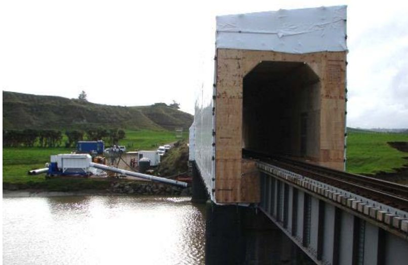
Figure 5.5: Full containment for repainting the Patea Rail Bridge
