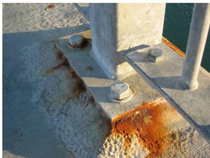
Figure 9.6: Unpainted galvanized base plate of handrail on coastal bridge
