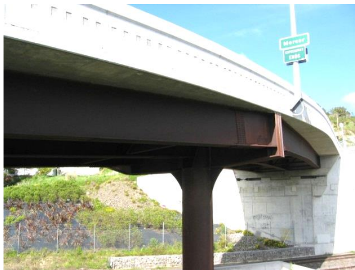
Figure 9.3: Mercer Bridge after four years weathering
