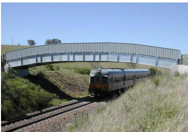
Figure 9.4: Example of a galvanized bridge
