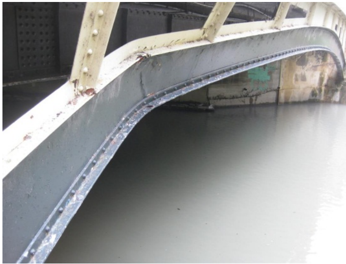
Figure 5.4: Example of damaged coatings – Auckland Harbour Bridge
