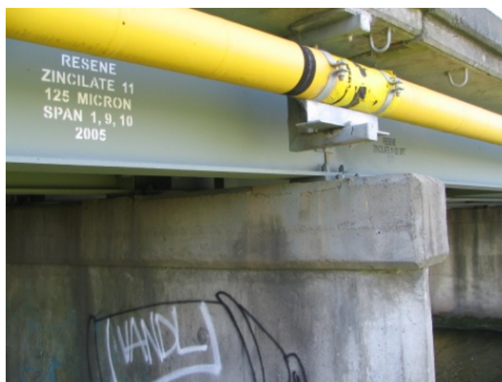
Figure 5.1: Example of stencilled repaint details on the Clive Bridge
