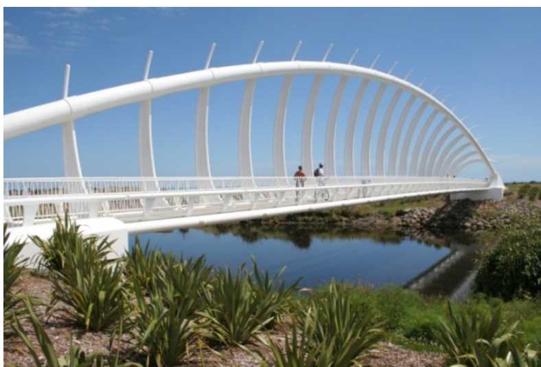
Figure 4.1: Example of coloured top coats on the international award winning Te Rewa Rewa foot bridge which was over 70% funded by the NZ Transport Agency
