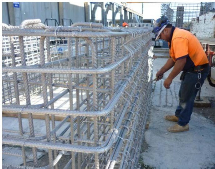
Figure 9.1: Wellington Harbour Culvert stainless steel reinforcement cage
