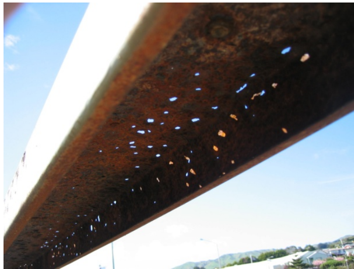
Figure 9.6: Unpainted galvanized base plate of handrail on coastal bridge
