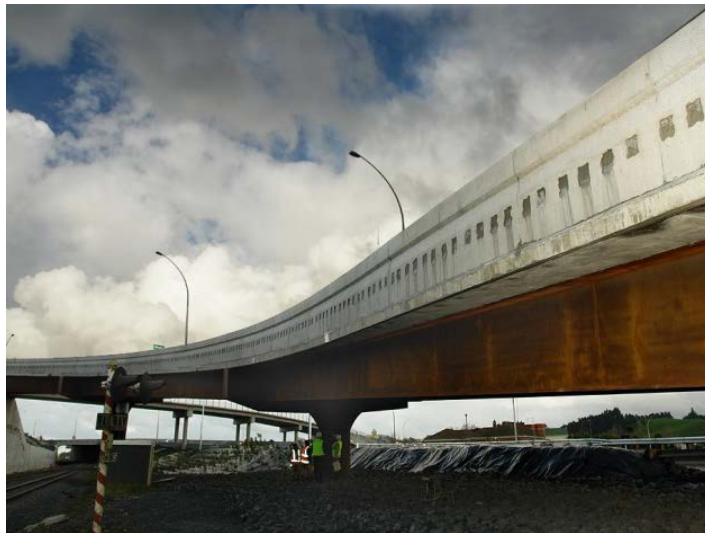
Figure 9.3: Mercer Bridge after four years weathering
