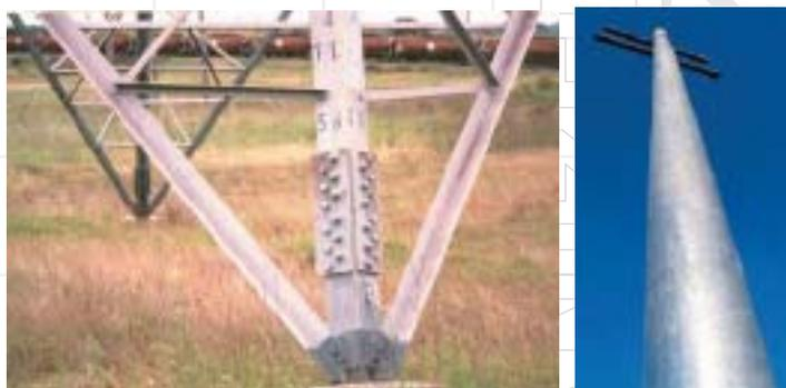
*The shape of a structure will have a significant impact on durability of the galvanized coating. The lattice tower has many overlap[ping joints and horizontal or upward facing surfaces. The galvanized monopole's surface is smooth and vertical. The galvanized coating on the pole will have at least 2X the life of that on the lattice tower.*
