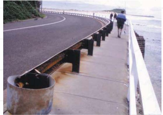
*Severe marine environments such as this ocean front site may have zinc corrosion rates of around 20 microns or more per year. In this environment, the galvanized coating on the guardrail has a predicted life of 3-5 years.*
