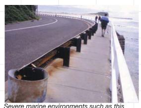
of around 20 microns or more per year. In this environment, the galvanized coating on the
