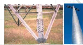
The shape of a structure will have a significant impact on durability of the galvanized coating. The lattice tower has many overlap[ping joints and horizontal or upward facing surfaces. The galvanized monopole's surface is smooth and vertical. The galvanized coating on the pole will have at least 2X the life of that on the lattice tower.
