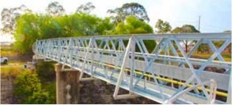
removed during the galvanizing process. This required the installation of temporary cross bracing inside the frames during transportation and lifting. The stabilising members were then bolted onto the outside of the truss prior to installation, and the temporary cross bracing was removed.
