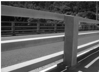
Figure 30 Wye River bridge rails and post with bolted base plate
