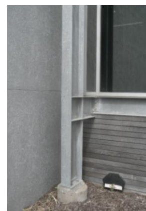
Figure 7 Structural beam exposed to the bay
