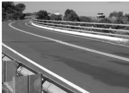
Figure 31 Kennett River bridge rails and safety barrier
