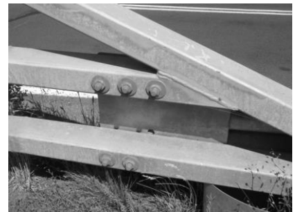
Figure 32 Bolted joints & welding before galvanizing in bridge rail
