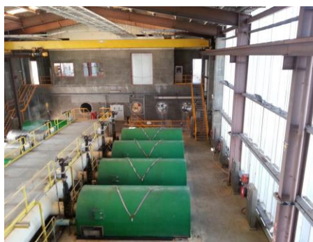
Figure 17 Fine screening building with duplex coated stairs and handrails
