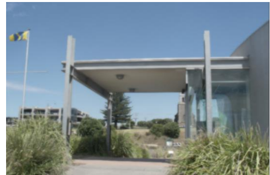
Figure 11 Hot dip galvanized beams hold up the entrance to the Centre
