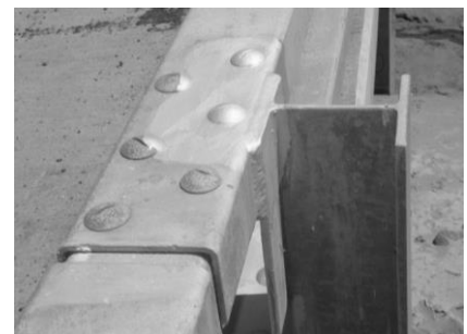
Figure 27 Repaired weld on bridge rail at Jamison River
