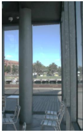
Figure 21 Corner of Pavilion showing hot dip galvanized column and mullions
