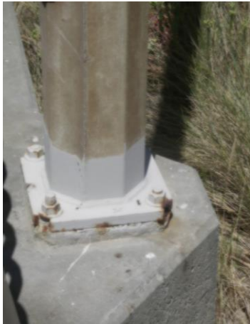
Figure 36 Painted bottom of lightly rusted, salt encrusted galvanized light pole
