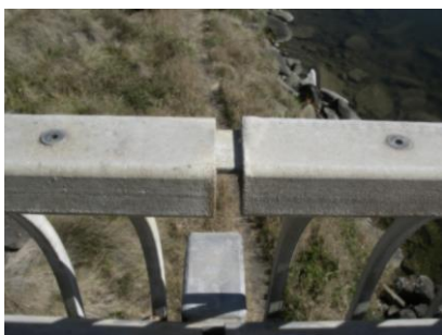
Figure 33 Symthe Creek bridge rail with salt encrusted galvanized coating
