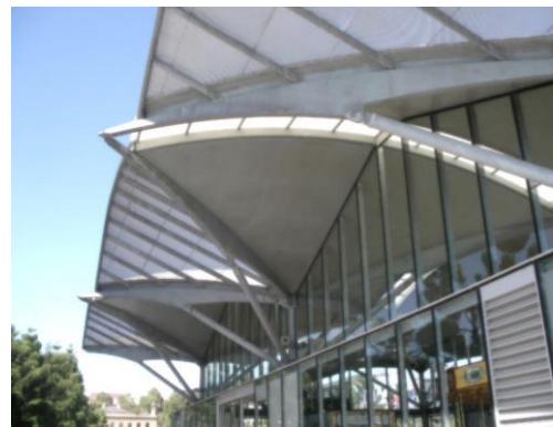
Figure 22 Curved roof of Pavilion with bolted joints
