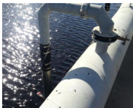
Figure 15 Neoprene sleeves separating hot dip galvanized pipe from immersed stainless steel pipe
