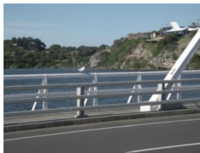
Figure 39 Duplex coated bridge rails at Hopkins River supports for footbridge
