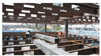
once again saving time and cost. The composite beams are bolted to 610 Universal edge beams, connected to the external steel diagrid via steel stub connections, which penetrate through the façade at regular grid spacings.
