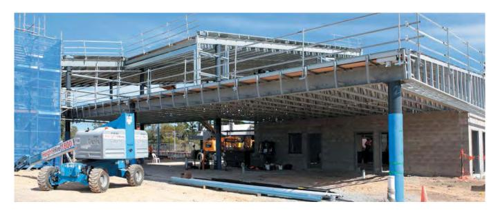
"For the braced bays, piles are required to resist the uplift due to the overturning induced by the lateral load on the building. The uplift values are too large to be resisted by reasonably sized pad footings."
