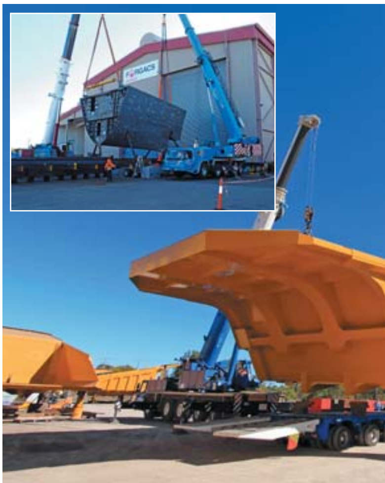
Inset: Turning of AWD block 113 in August 2012 at Forgacs Shipyard Newcastle
