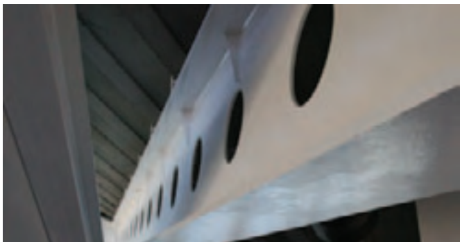
Long span welded steel beams 1,000 millimetre deep dominating the concourse. Castellated style penetrations have been cut into the beams to lighten the visual impact.
