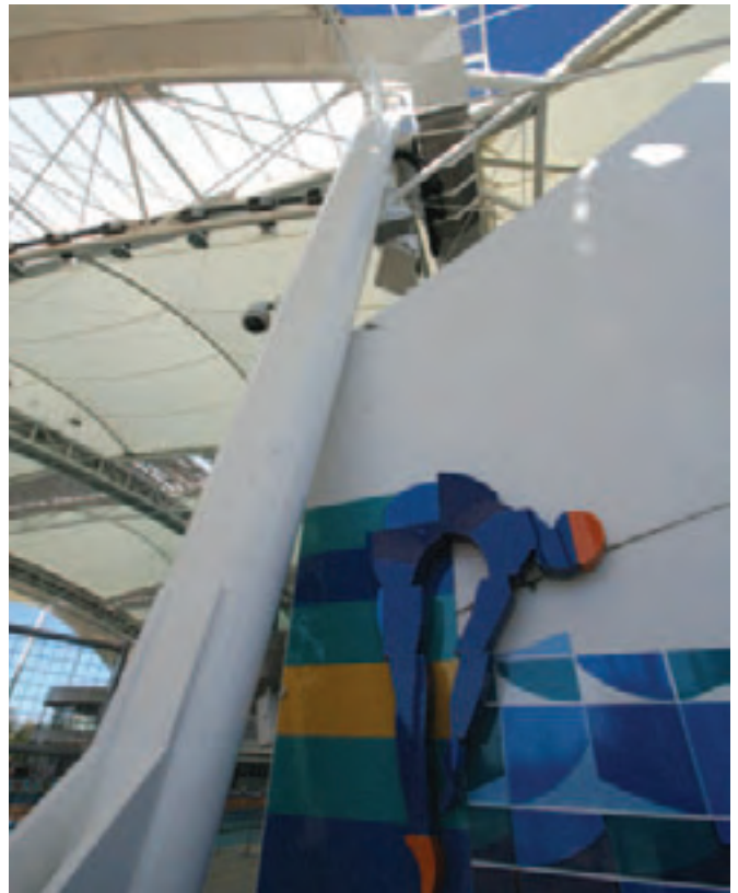
Slender cigar shaped tapered columns were connected to the roof structure at a third of their height.
