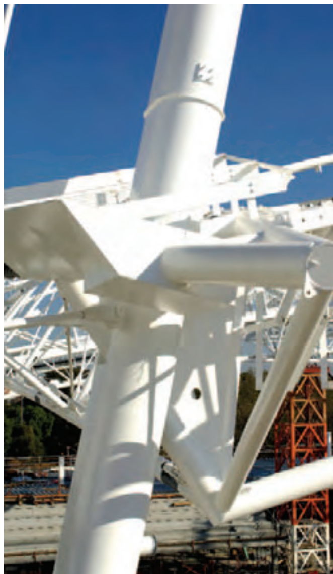
Pinned connections were adopted at the base of each mast and at each "knuckle joint" connection to the roof trusses in order to minimise bending action in the masts.
