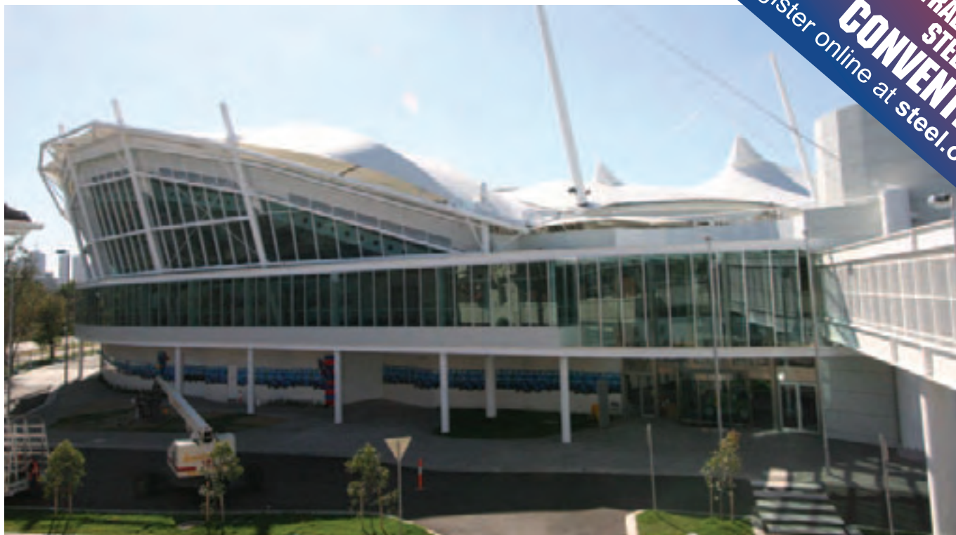
Expressed steel and glass facade at the entrance to Stage 2. Cable stays connecting the new structure to the existing building can be seen.
