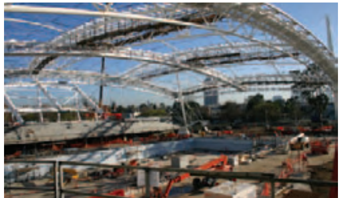
The permanent frame of the pool roof is supported by four space-trusses, to which the grandstand roof is attached on the west and the temporary roofs on the north and west.
