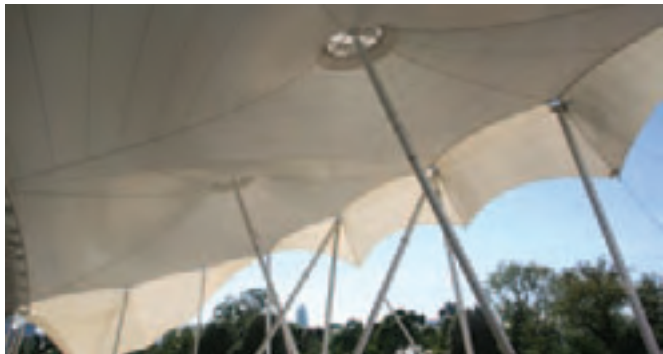
The temporary roof has a different fabric for economy and speed of erection/dismantling. They have conical forms with internal push-up masts and parametre mast catenary cable supports.
