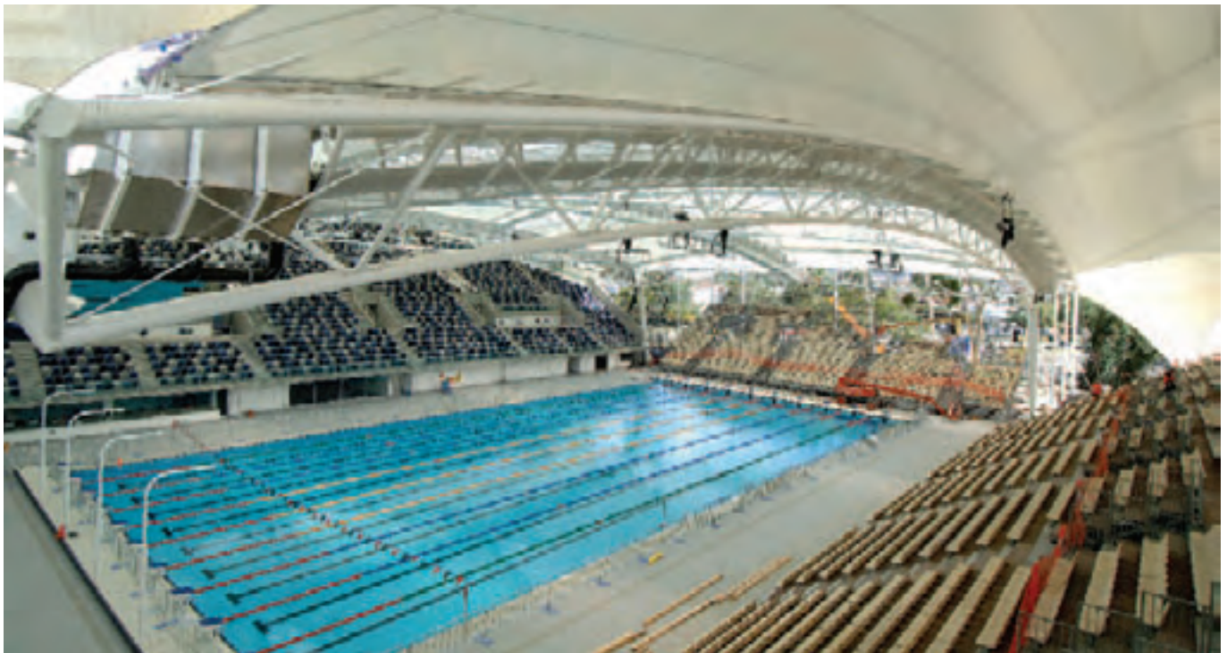
A cable stayed steel frame of the pool roof spans 70 metres and supports three tensioned fabric panels. Temporary seating is to the right and centre.
