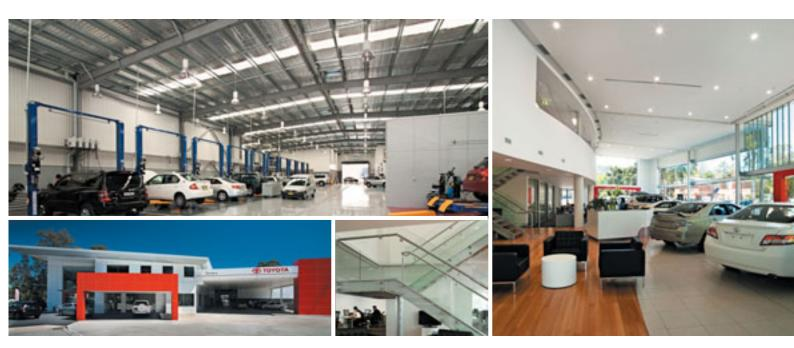
"However, the deployment of tall portal frames with slender members presented a challenge in controlling deflection so slender steel columns up to 12m centres were used to reduce the impact of the structure.
