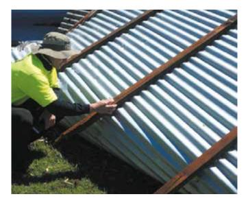
Previous investigations following severe wind events have found that flashings fastened with pop rivets have often detached from buildings. Flashings that were fastened with screws on all sides performed well. In a few buildings assessed during the investigation, loss of flashings contributed to partial loss of the adjacent roof sheeting.
