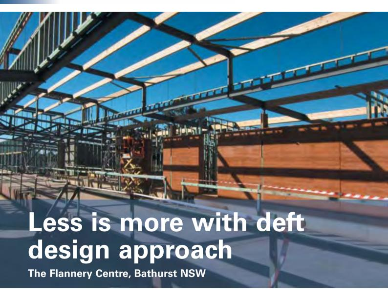
The decision by structural engineers, Northrop Engineers to substitute steel portal frames with a braced frame structure in planning a new green skills centre in regional NSW provided a 35 percent saving in steel tonnage to help the building attain its targeted 6-Star Green Star rating.
