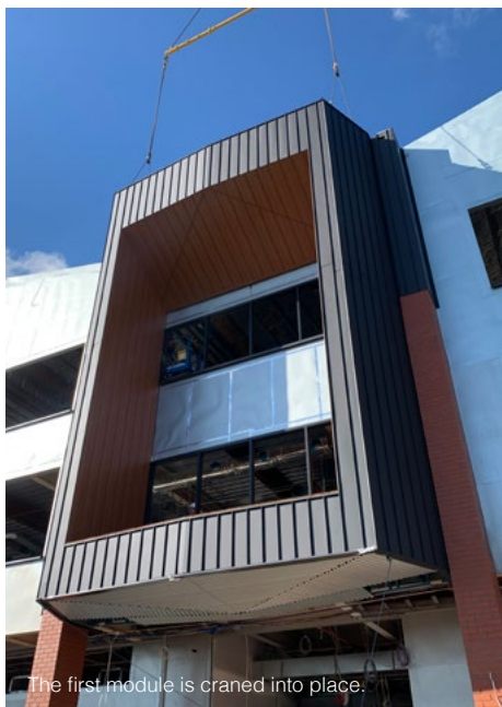
More modules are erected on-site.
