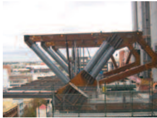
The success of the Latitude@ World Square construction process hinges on these huge "jump start" trusses, effective in large part due to the light weight and great strength of Bisplate 80.
