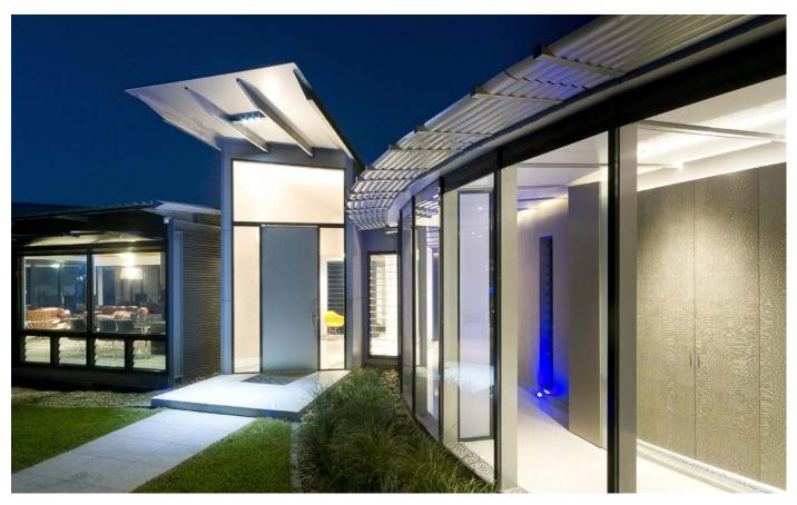
The extensive use of steel in the design allowed the builder and architect to closely control costs by maximising off-site prefabrication of building elements. Steel components were procured well in advance under fixed price orders and careful detailing ensured minimum rework. Site installation was rapid and required minimum labour and relatively small cranes.
