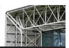
The Sainsbury Centre for the Performing Arts was designed and constructed by Norman Foster in 1977. The British High Tech movement brought exposed structural steel to the forefront of design, and with it an array of issues that had not a been part of architectural discourse for more than a century. The project used CHS members and a structure that was expressed on the exterior and interior of the building.
