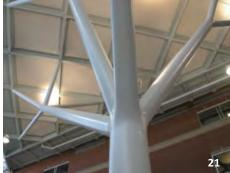
Two different steel trees. One created using I shapes to create a very textured appearance, the other using mechanical pipe and specialty castings and striving for a seamless appearance, using a high gloss finish. AESS specifications must be tailored to the overall design intentions of each individual project as they are all somewhat unique.
