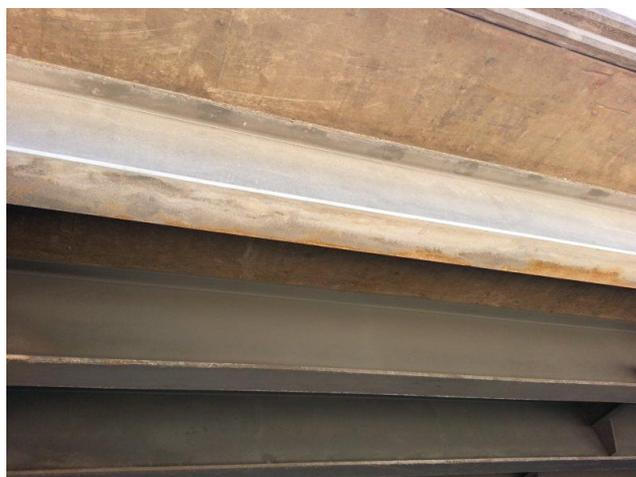
Figure 6: Overcoating trial at Graham Street overpass.
