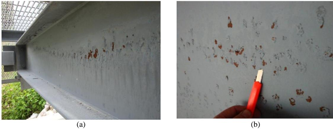
Figure 4: Spot rusting and blistering on WB-IZS coating from alkali production as a result of condensation during curing (8)
