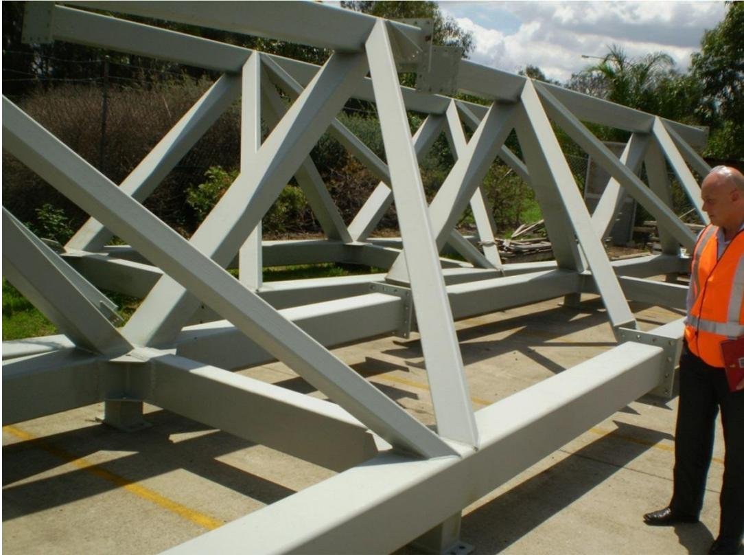
Figure 2: The non-compliant steel truss
