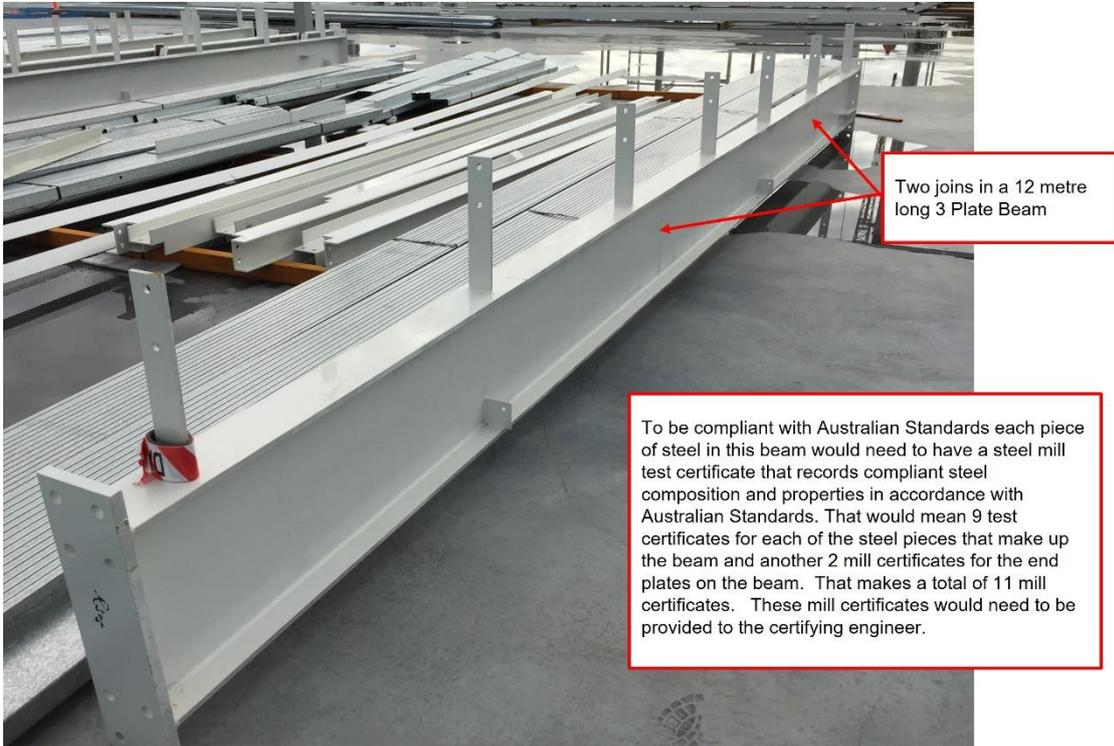
Figure 10: Imported welded 3 plate beams – extra joins increase risk of non-compliance
