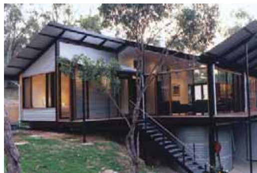
Zincalume roof and wall cladding distinguish this bush house.
