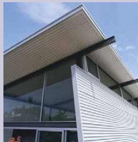
Steel on the roof, eaves and a feature blade wall create a striking split-level townhouse.
