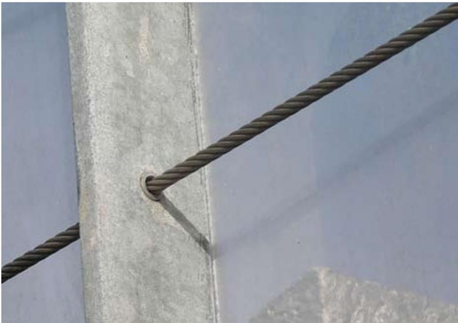
Prevention of bimetallic corrosion in a highly corrosive coastal environment. The stainless steel wire is electrically isolated from the hot dip galvanized balustrade.
