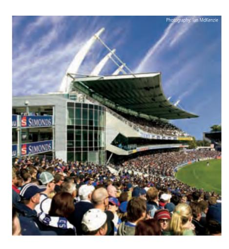
Stadium with Peddle Thorp, we knew that steel is the best material to support the cantilevering seating tiers. So we had major steel elements in the front seating areas, at the rear with the major masts, and over the top with the upper deck and roof. Because the site was so tight, it quickly became obvious that a steel frame was the best solution."
