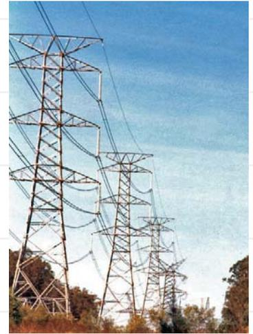
*Galvanized steel structures such as these transmission towers have a long service life exceeding 50 years and are 100% recyclable. In addition, the steel could be re-galvanized for a minimal energy cost to preserve the steel indefinitely.*
