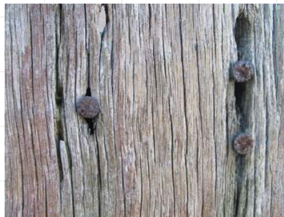
Uncoated steel nails used in hardwood not only corrode themselves by the corrosion products attach the surrounding timber
