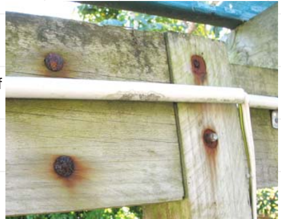
CCA treated pine is very aggressive on both zinc and steel when its moisture content exceeds 20%. These electroplated bolts have almost totally corroded in pergola structure after 10 years.
