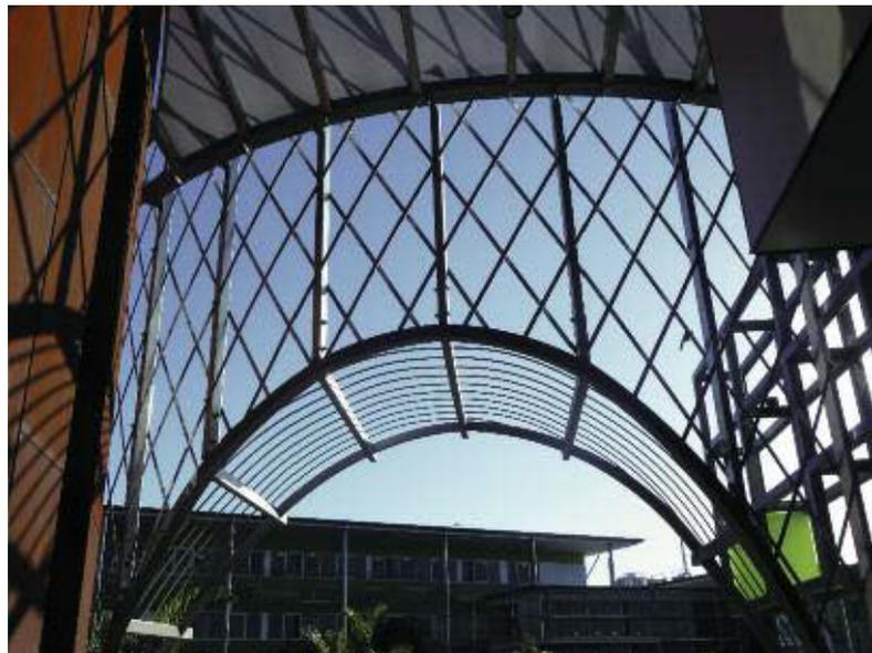
Mr Kenny said a defining aspect of the Cairns Institute is the knowledge wall which effectively cuts the building in half and cantilevers 7.2 out of each end of the complex. The knowledge wall consists of two modular, welded frames 0.8m apart and welded together at regular nodes to provide a 'box' like structure. The structure is penetrated randomly to support cantilevering rooms and offices.
