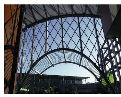
Mr Kenny said a defining aspect of the Cairns Institute is the knowledge wall which effectively cuts the building in half and cantilevers 7.2 out of each end of the complex. The knowledge wall consists of two modular, welded frames 0.8m apart and welded together at regular nodes to provide a 'box' like structure. The structure is penetrated randomly to support cantilevering rooms and offices.
