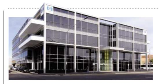
THE BUILT ENVIRONS DEVELOPMENT, LOCATED AT THE CORNER OF FROME AND FLINDERS STREETS IN ADELAIDE, SOUTH AUSTRALIA, PROVIDES CAR PARKING IN A BASEMENT, PLUS 4 LEVELS (EACH 1280M<sup>2</sup>) OF OFFICE CONSTRUCTION WITH A PLANT ROOM ABOVE.
