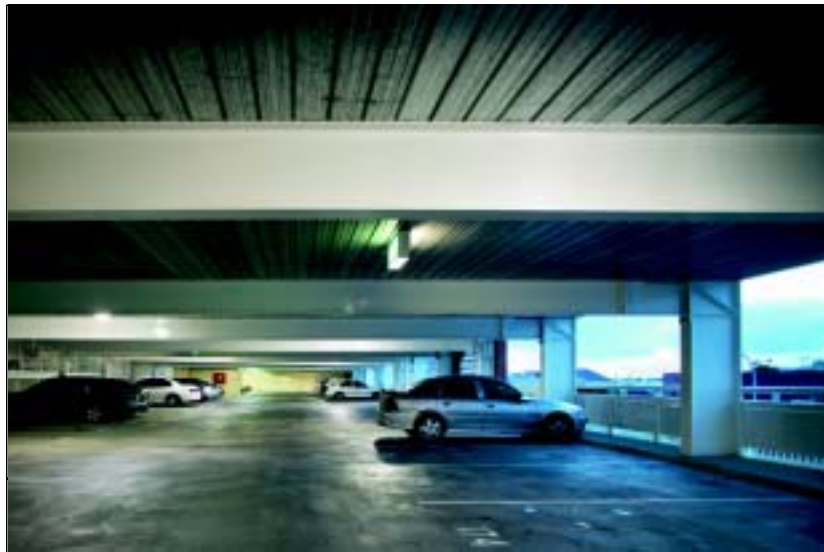
carpark with bare steel beams and columns
