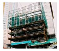
All primary and secondary steel beams are unprotected throughout the building, with the exception of beams passing through the atrium. All columns and transfer beams are protected in accordance with DTS, ie 120/-/- FRL in offices and 180/-/- FRL in retail spaces.
